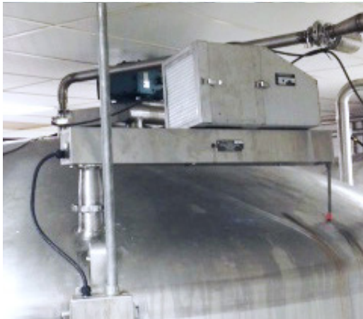
Custom LTC Installation with additional heater element
